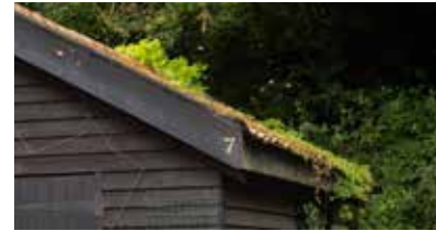
Tiled roof and timber weatherboarding
