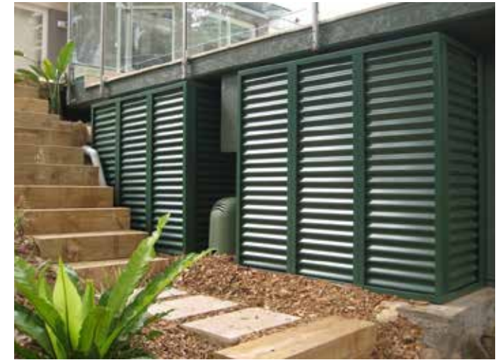
Figure 72: Concealed tanks integrated with the design.
