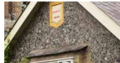
Flint on a building facade
