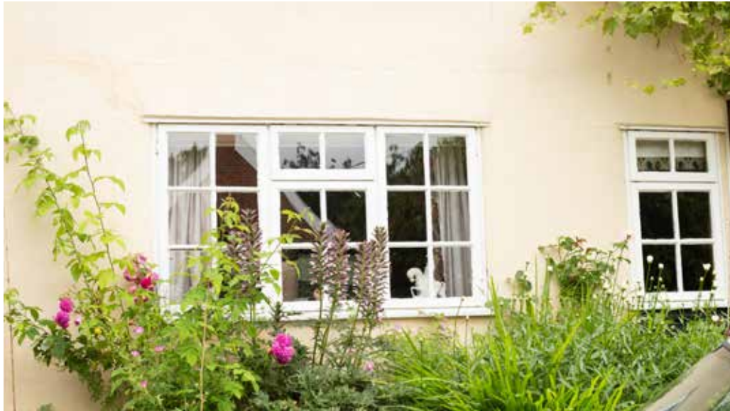
Figure 33: Local example of sashed windows within the conservation area, Low Street.
