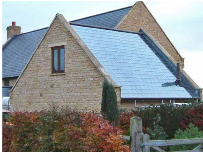
Figure 71: Retrofitted solar panels integrated sympathetically with a traditional building.
