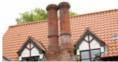
Strong chimney, dormer and clay tiles
