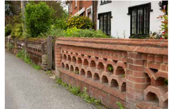
Banham bricks on property boundary.
