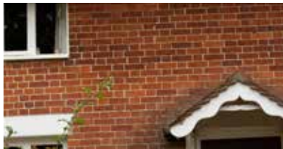
Brick timber window frames and wood detailing
