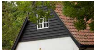
Subtle combination of materials. Weatherboarding, render and tiles
