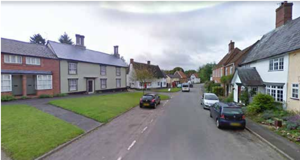
Figure 12: Local example of street typology 5, Low Street.
