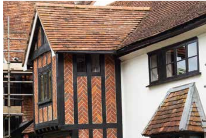
Plaintile on roofs and brick nogging on walls.
