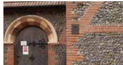
Flint and brick detailing on community hall
